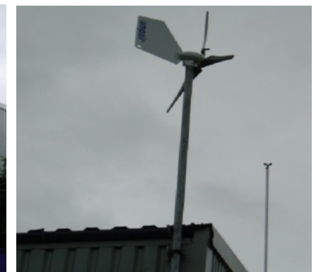
Figure 2. The average power generated by this Ampair 600-W micro-turbine in Leamington Spa is 0.037 kWh per day (1.5 W). For comparison, the average British person's share of electricity consumption is 17 kWh per day.
