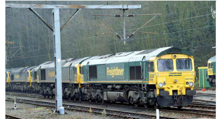
Figure 1. A diesel freight train running on an electrified track. Photo: © railway-technology.com.
