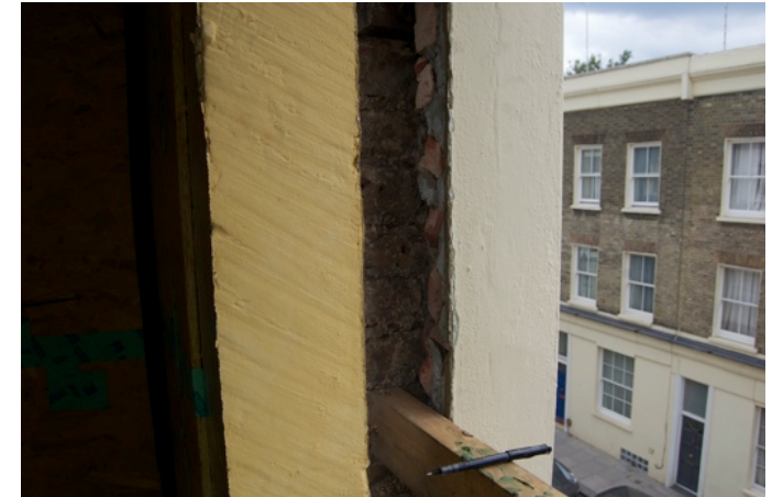
Figure 1. Internal solid wall insulation in a London home being enhanced as part of Retrofit for the Future.
