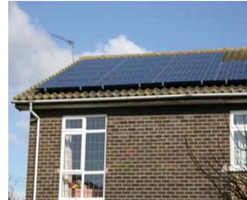
Figure 1. The peak power delivered by this 25 m 2 array is about 4 kW. The average is 0.5 kW, equivalent to 20 W/m 2 .
